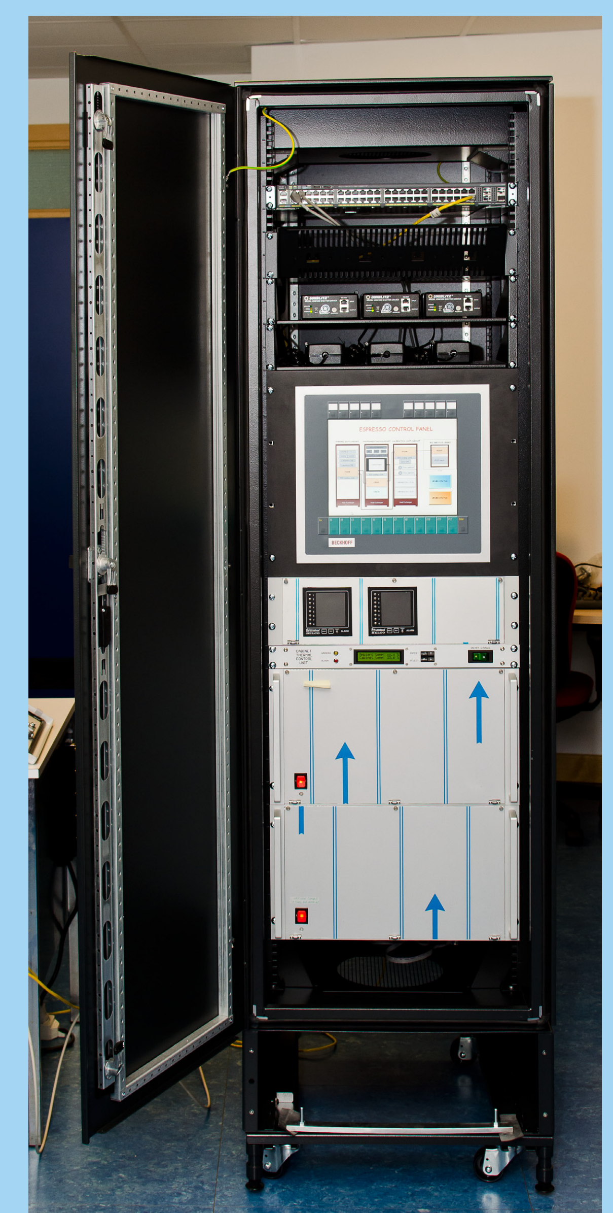
Figure 5 ESPRESSO instrument main cabinet
